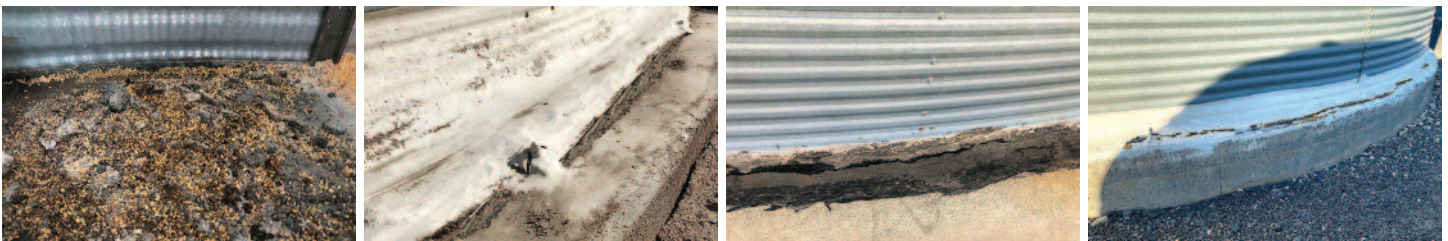
Bins expand and contract. Sealants crack and leak. Grain rots, bins rust & bugs thrive.
